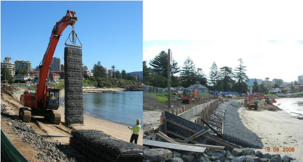
Triton ® mattresses being installed
