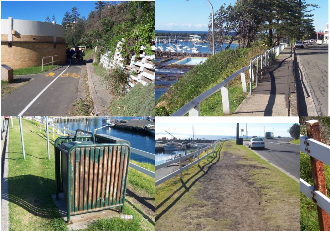
Examples of dilapidated infrastructure
